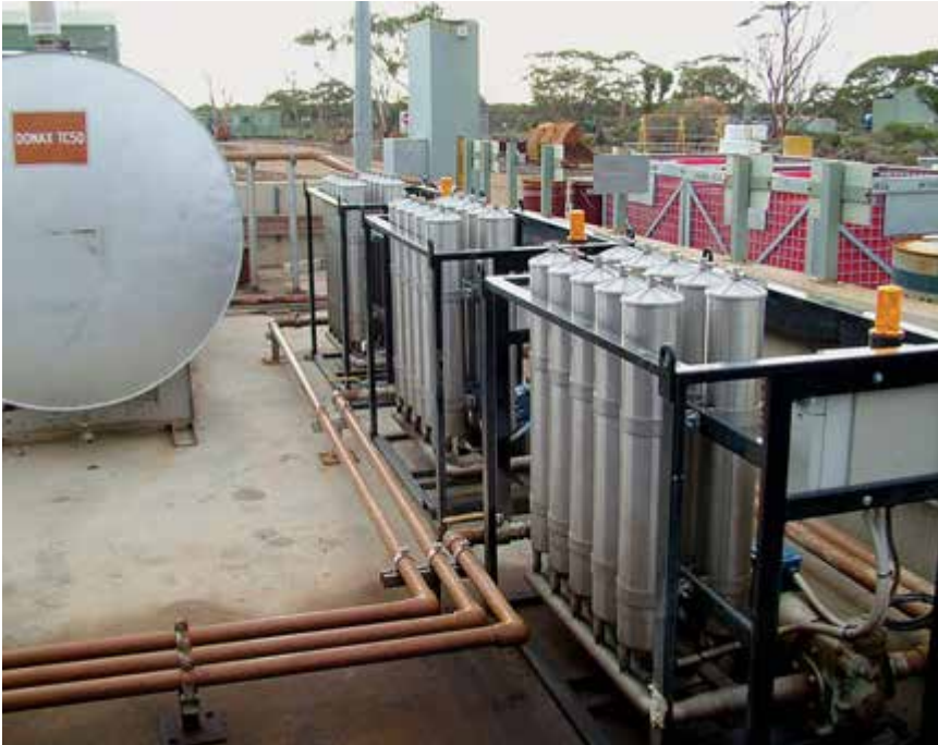
Bulk fuel filtration systems prevent contaminants from entering vehicles' fuel systems, improving reliability and performance, as well as reducing wear and breakdowns.
